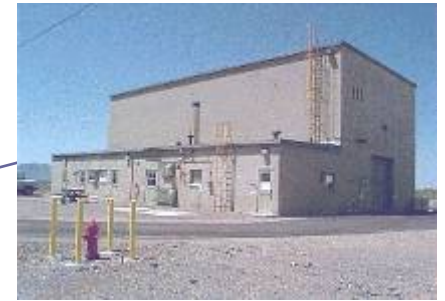
Contraband Test Bed
