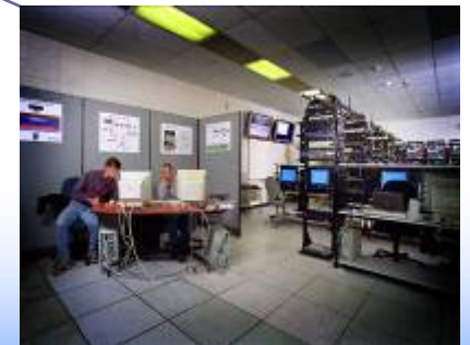
SCADA Test Bed
